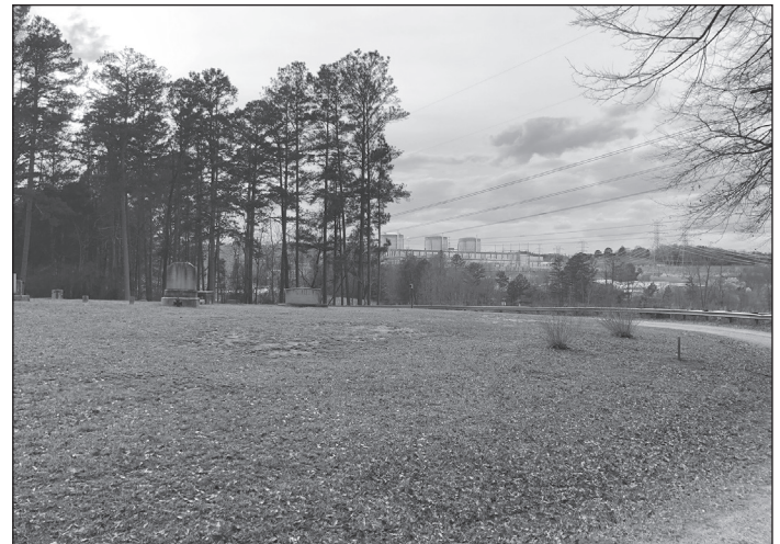
Old Pickens Presbyterian Church graveyard in foreground with Oconee Nuclear Site's three 1974-vintage Babcock & Wilcox pressurized water reactors in the background. The three Duke Power reactors do not have cooling towers — they dump boiling hot water directly into Lake Keowee. Photo: Joanne Steele, 2020
